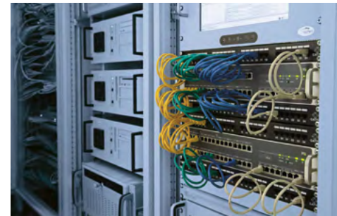
INTUS ACM80e Rack with patch panel
